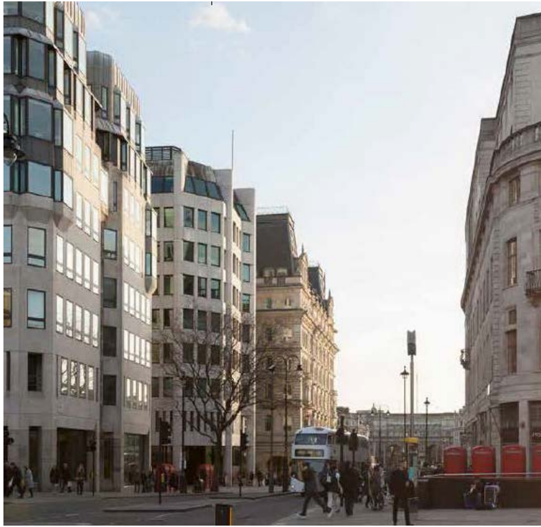
Existing view from Strand
