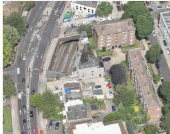
View of railway cutting (top) and aerial view of site looking south (bottom left) and aerial view of site looking north (bottom right).
